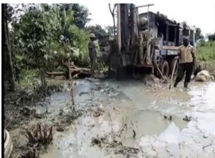
Heavy drilling equipment trying to cross the small river.
